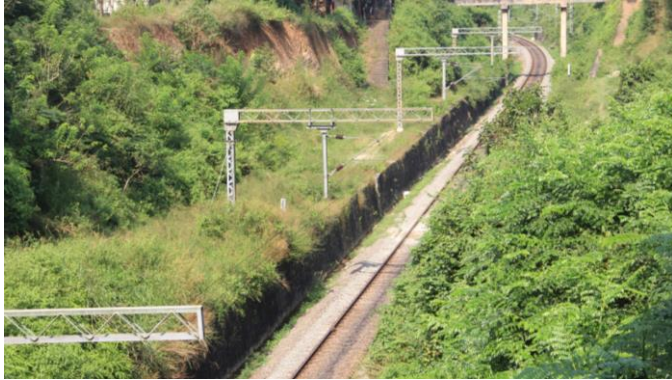
Figure 30: Kuzhithurai Railway Station
